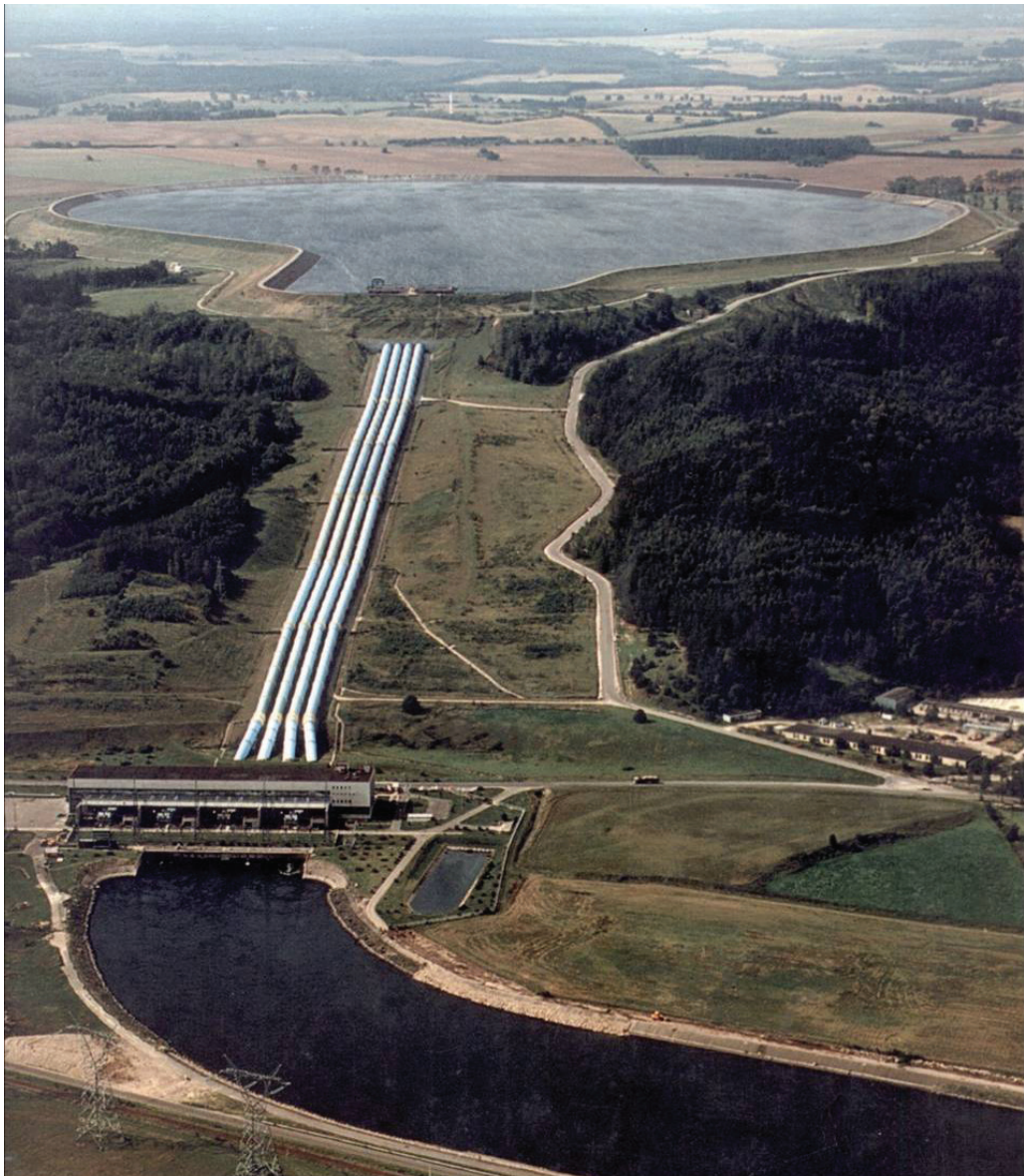
Fig. 1. Aerial view of Żarnowiec hydropower plant (Brochure, 1998)
